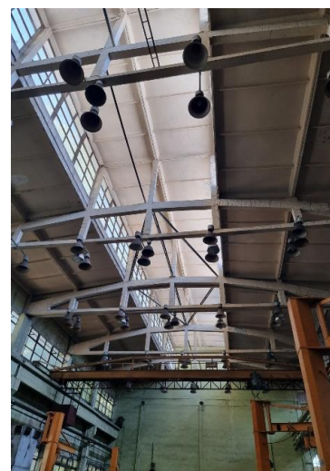
Old conventional lighting in the production premises
