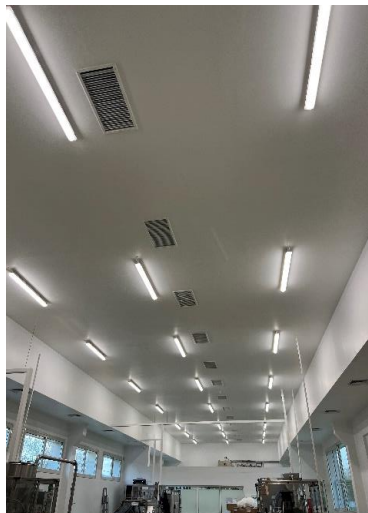
New lighting in the production premises
