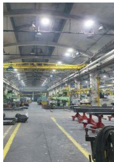
Old conventional lighting in the production premises
