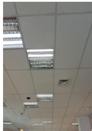
Old conventional lighting in the production premises
