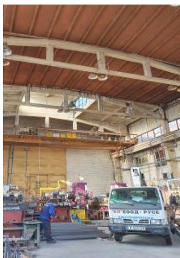
Old conventional lighting in the production premises
