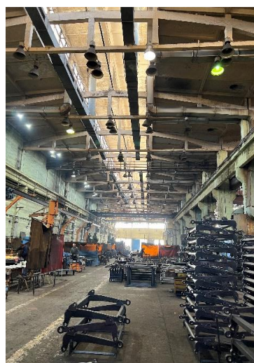
Old conventional lighting in the production premises
